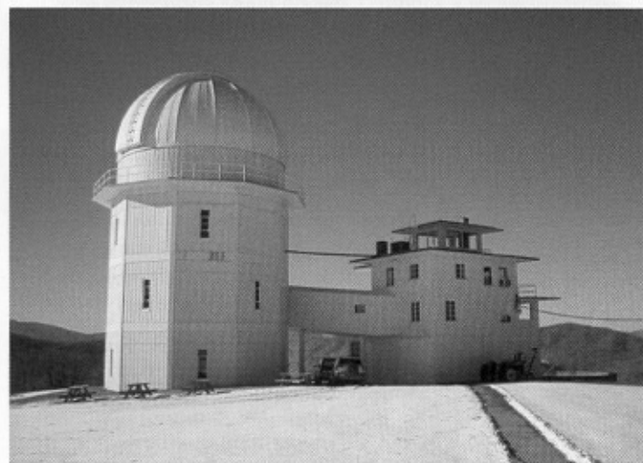
The main observatory building and the dome of the 40-inch telescope.
